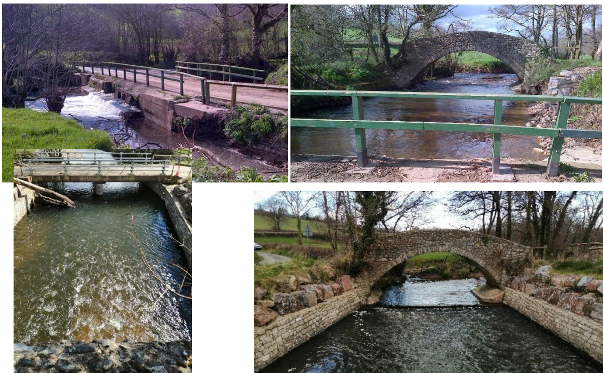
Figure 40: Alterations at Beckford Bridge affecting bed levels and fish passage
