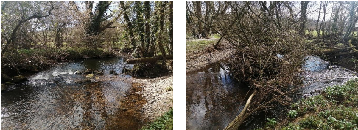
Figure 36: former bed and bank protection measures are failing as they are undermined, even large tree jams are unable on their own to stop the erosion processes entirely
