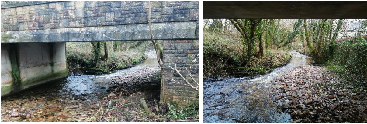
Figure 7: left hand side berm might be removed, and the bed reinforced with large stone size mix
