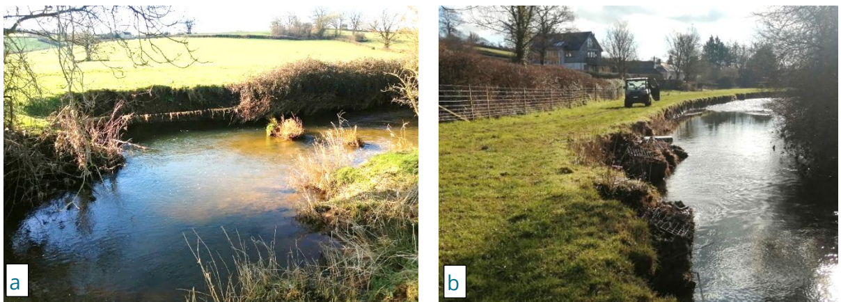
Figure 23: a) Erosion starting on right bank in response to lowering bed levels downstream, b) erosion to the left downstream exposing and undermining old bank protection.
