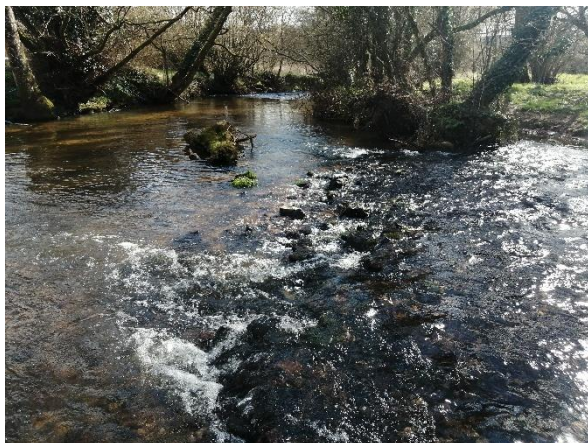
Figure 34: A weir formed of oversized stone holds the bed intact upstream, whereas downstream the deepened channel is smothered in fine sediments
