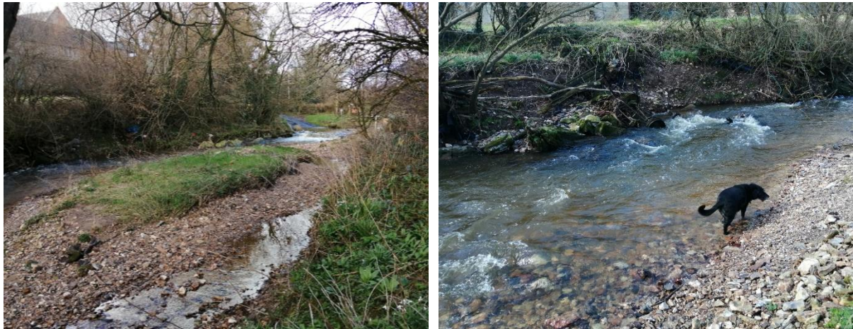
Figure 14: Flows pass over the pipe ford, with flows and bed incision concentrated on the western side
