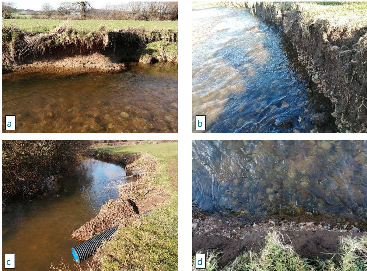
Figure 20: Bed incision a) upstream 150m with silted bed, b) limited shallow incision below first meander, c) undermining former gabion bank protection, d) incision dropping below gravel strata
