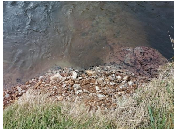
Figure 15: Upstream left bank erosion; the banks are formed of terrace fill above underlying clay geology layer
